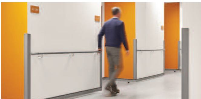
Handrails were installed in the corridors at the Grange University Hospital, to offer patients support and respite, protecting them against falls, and also safeguarding their health and dignity.
